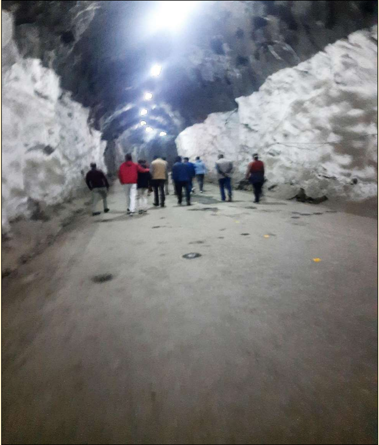
Main Access Tunnel to the 480 MW URI HEC Project
